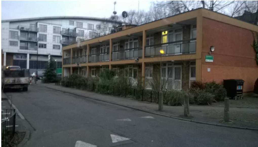
View from Hungerford Road looking west
