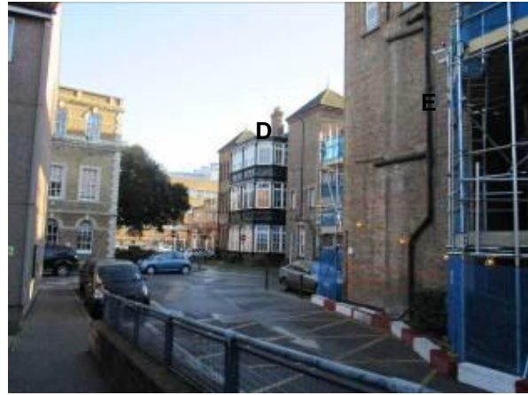
(looking South East)
